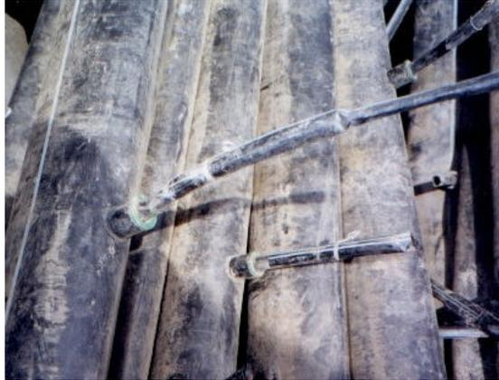
Figure 3. Manifold connection with punched socket fitting, a short section of polyethylene hose and wire ties to the tape.
